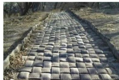
(f) Well-paved road using waste tyres [113]
